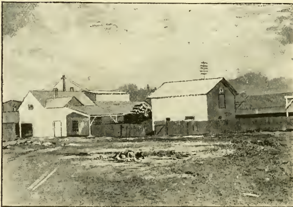
Coal and Wood Yards, Waterbury—W. H. Scott & Co.
